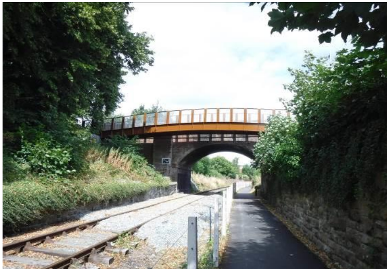
Lys Lane Footbridge – Bridge Replacement
